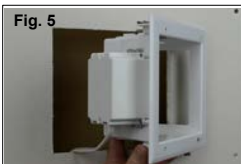
Figure 5: Use the four provided screws to secure the Old Work Electrical Box and Receptacle to the mounting studs on the back side of the Expandable Media Box.
